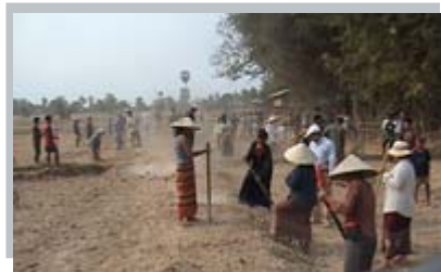
Villagers and PRF staffs helping while rural roads are being repaired
