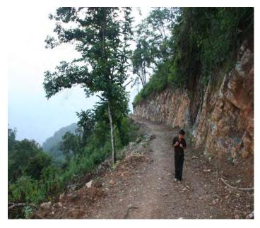
Because of the above constraints earth works are hampered by rocks and dynamiting the rocks is causing extra work and costs. In the case of Nong Het Tai road the cost for dynamiting rock was not calculated but put as a burden to the villagers.
